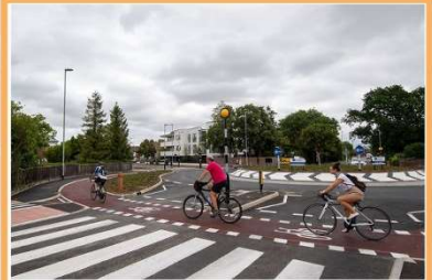
A Dutch-style roundabout is designed to create a safer environment for people walking and cycling by providing a formal crossing point at each arm of the roundabout.
